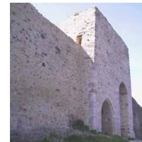
The iron door, secondary entrance of the castle.
