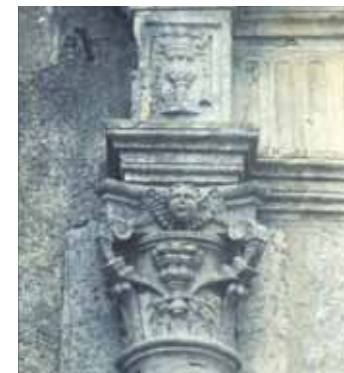
Detail of the porch of the church.
